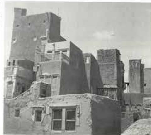
7.1, 7.2 and 7.3 Townhouses and wind-catchers, Thatta. Thatta presents a rare combination of urban verticality with rustic wattle and dash surfaces. On every roof is perched a wind-catching device, known locally as a "mangh".
