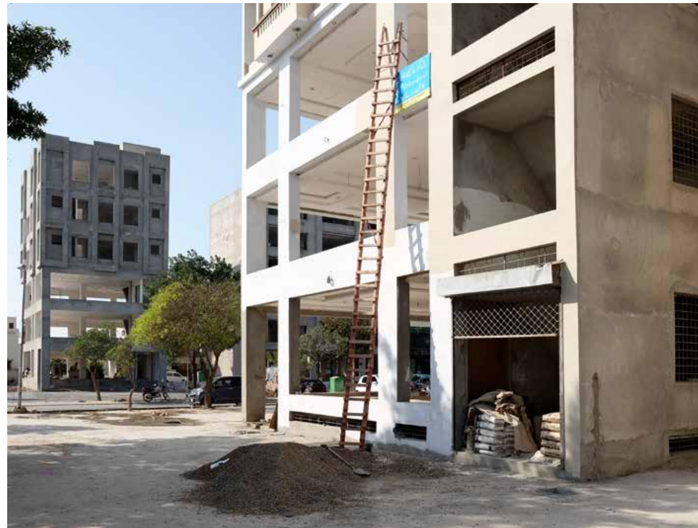
11.1 Construction in Bahria Town, Lahore, 2018. Image by Chris Moffat.
