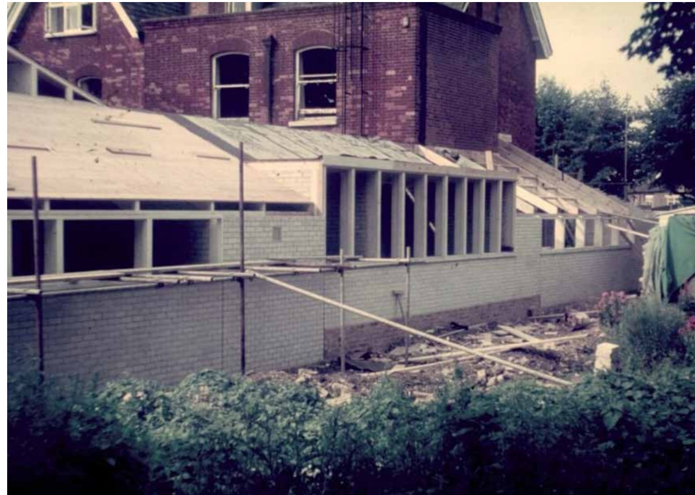
2.4 Children's Clinic under construction in Bromley, Kent, by Architects Co-Partnership, 1964.
