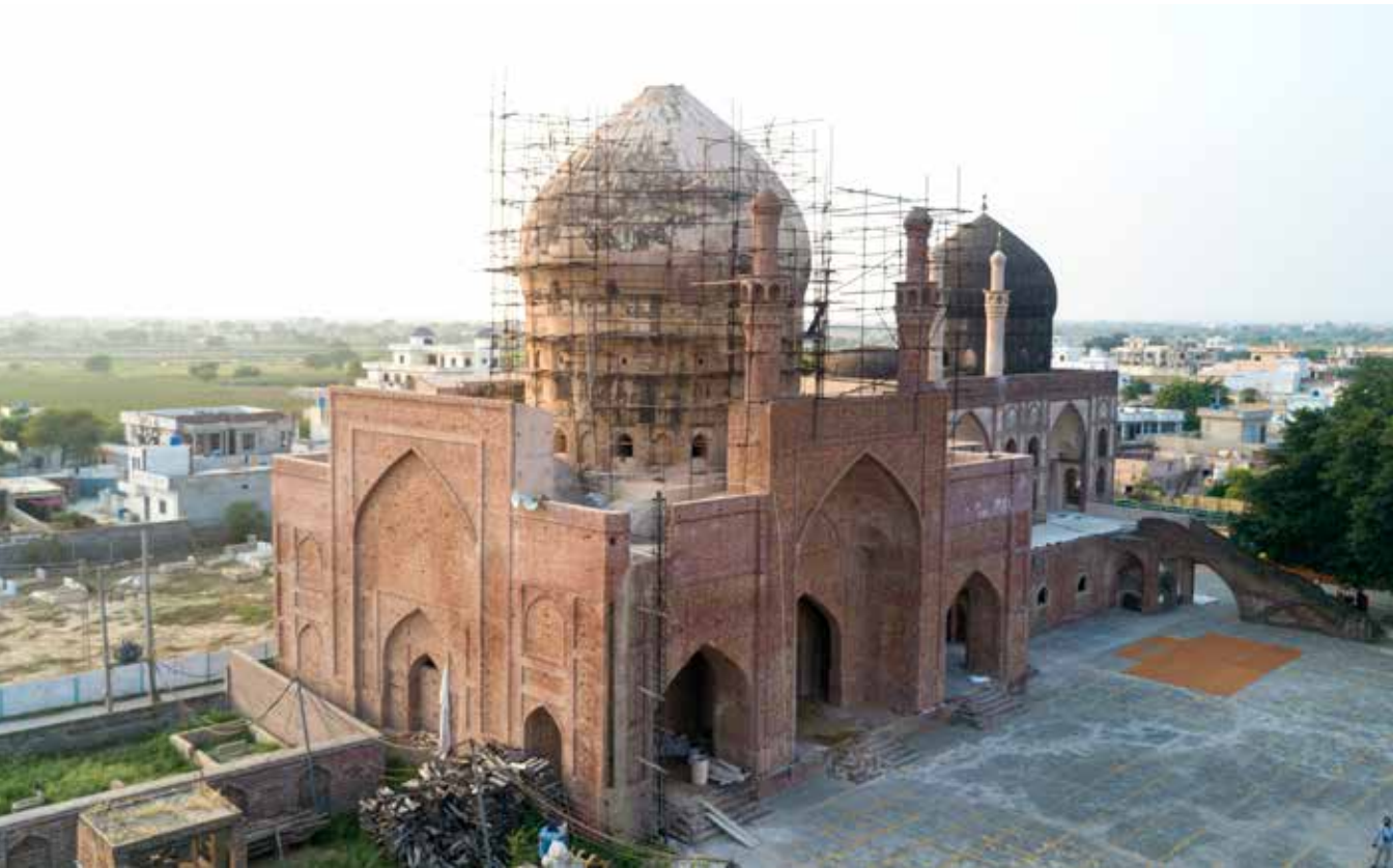
0.4 Construction of Challe Sharif Tomb and Mosque, Gujrat, 2022. Courtesy: RK Studios.
