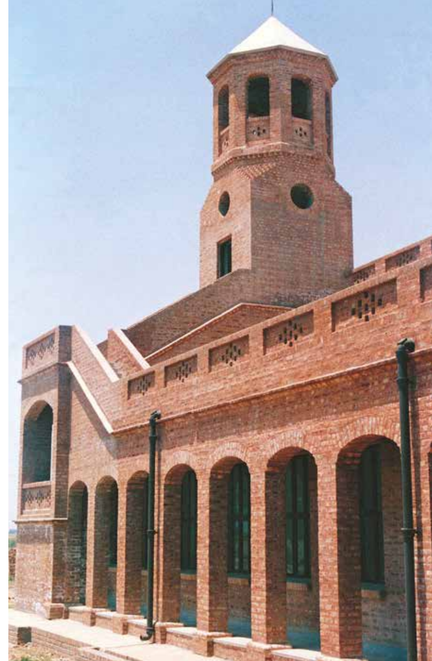
7.7 Administrative Block, Chand Bagh School, Muridke, 1994.
