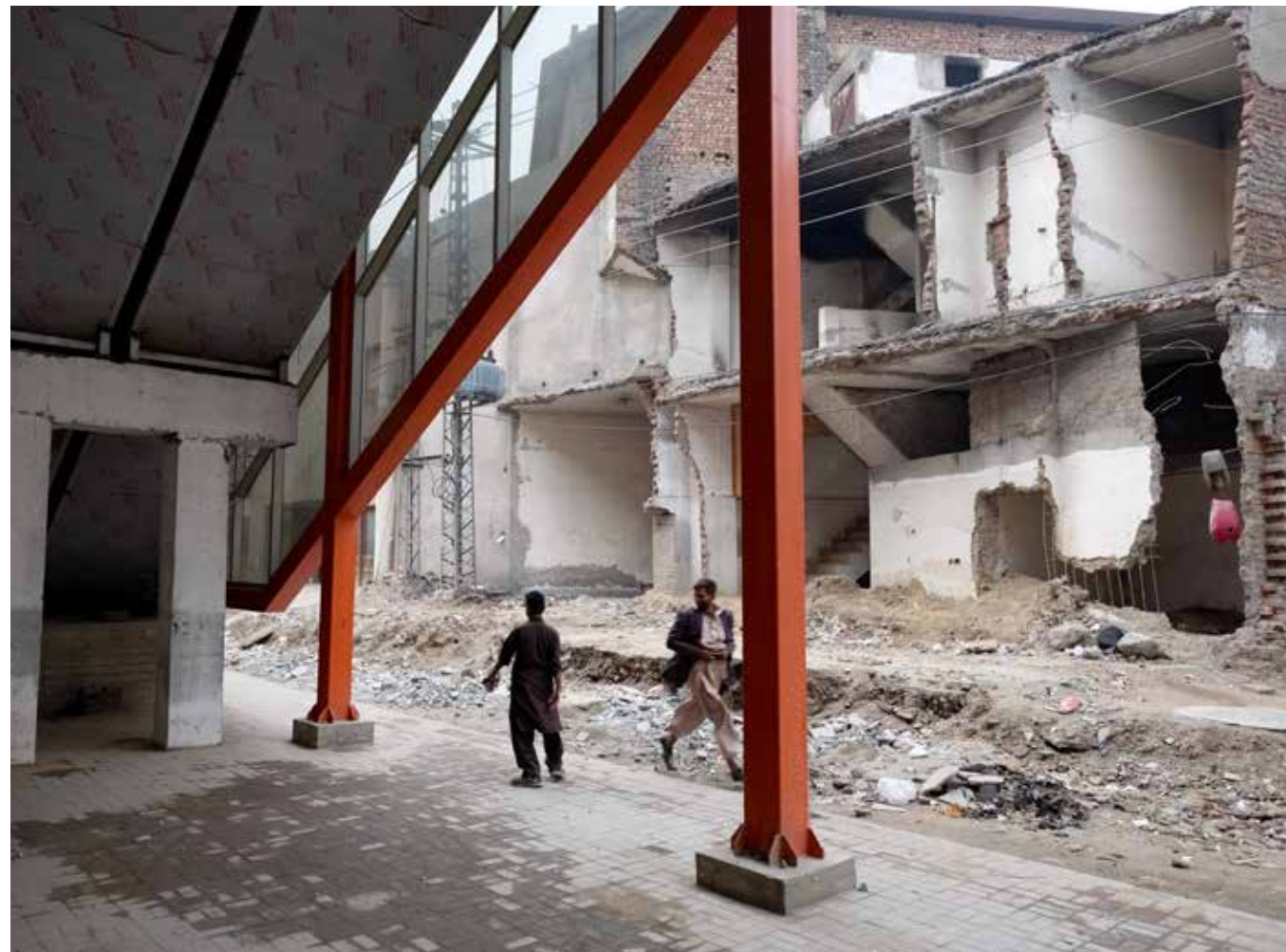
10.4 Construction of Orange Line, Lahore, 2019. Image by Chris Moffat.
