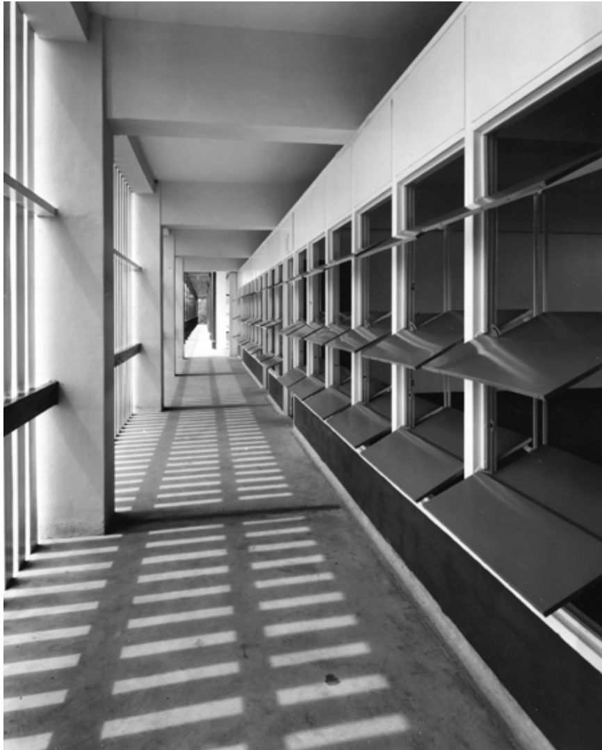
3.1 Lecture Room Block at KNUST, Kumasi. James Cubitt & Partners, 1956. Courtesy: Architectural Press Archives, RIBA.
