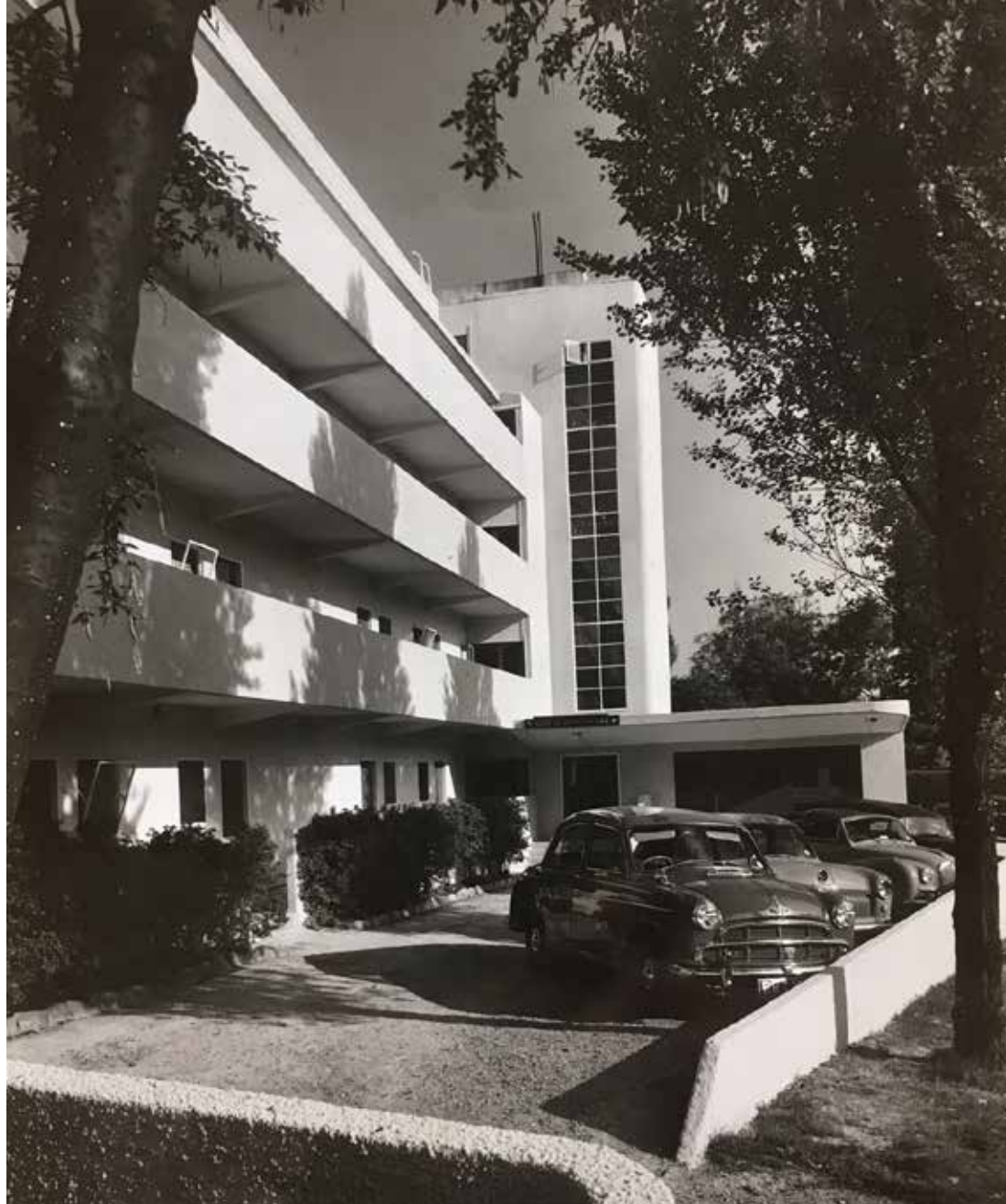
1.4 The Isokon Building on Lawn Road, Belsize Park, London in the 1950s. Courtesy: Pritchard Papers, University of East Anglia.
