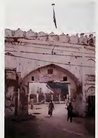
Hyderabad fort. The old fort door has been moved inside the city walls.
