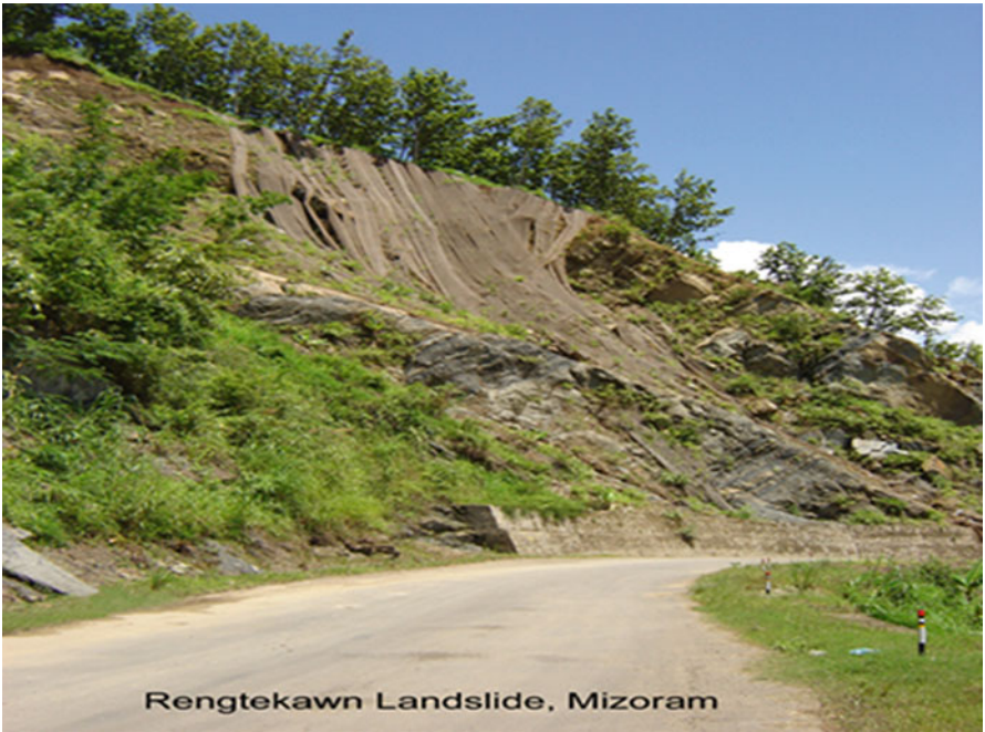
Photo 7.2 The Rengtekawn landslide, Mizoram (Photo Dr. R P Tiwari)
