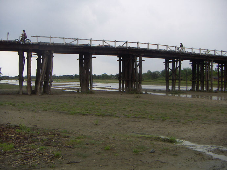
Photo 18.1 A timber bridge, use of wooden pillars as columns, north of Brahmaputra, Eastern Assam (Photo S. R. Jog)
