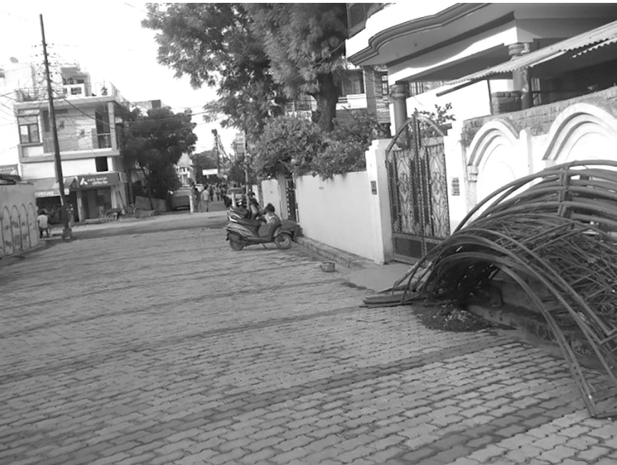
Figure 8.3 Renovated 26 A B with the original red stone pillars
