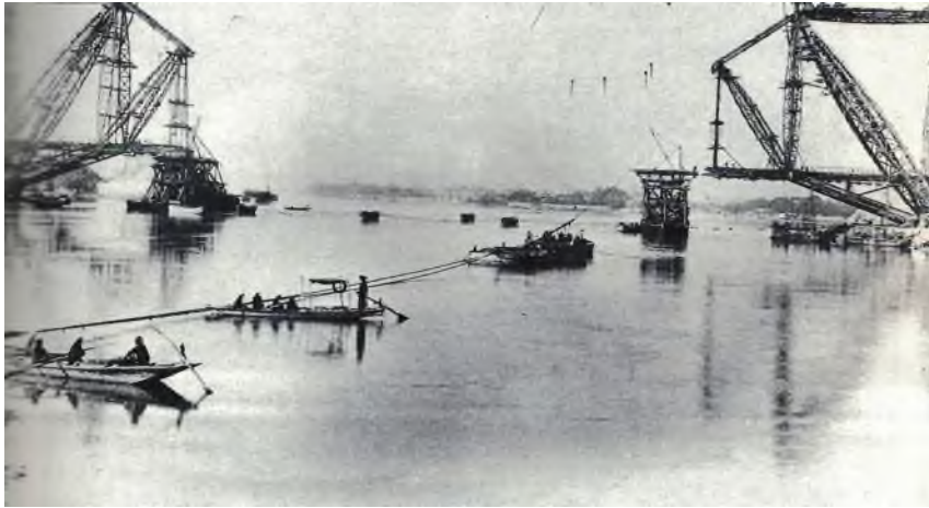
The Raj, c. 1895. Bridge under construction on the Indus at Sukkur.
