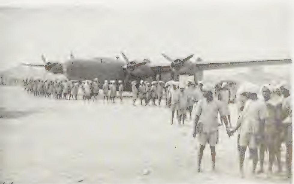
7. Building a US Army Air Force Base in Assam, c. 1943
