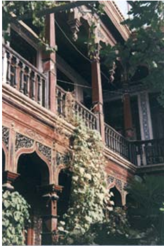
FIG. 22. Kashghar. Decorated balustrade. (Photo: Courtesy of R. G. Rozi.)
