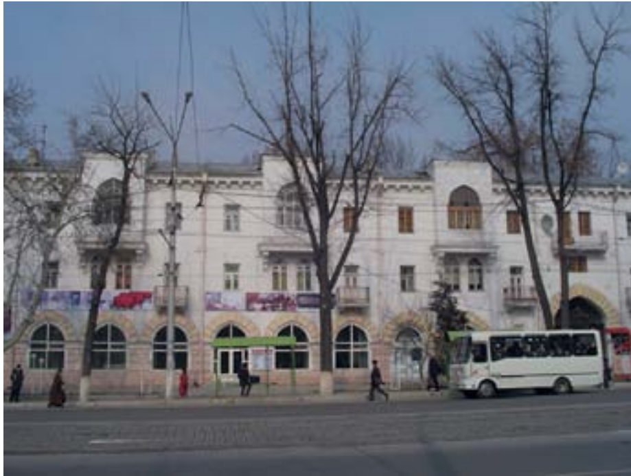
FIG. 7. Tashkent. Apartments on Navoi Avenue. 1949–50. Architects: M. Bulatov and L. Karash. (Photo: Courtesy of M. Azzout and G. Akramova.)
