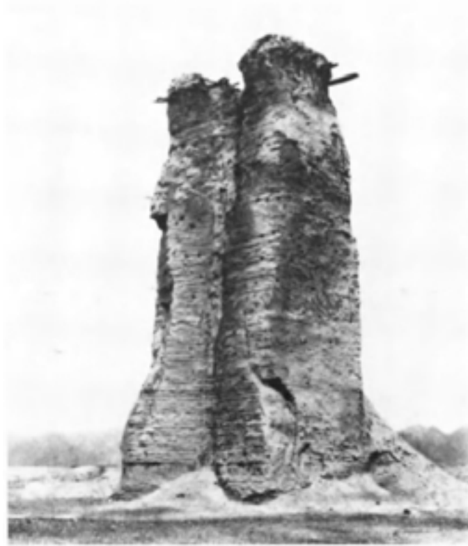
FIG. 12. Remains of a Han beacon tower.
