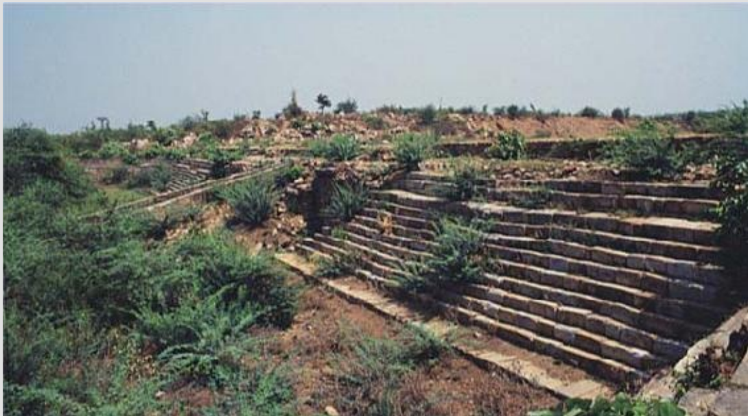
THE ANANGPUR DAM
