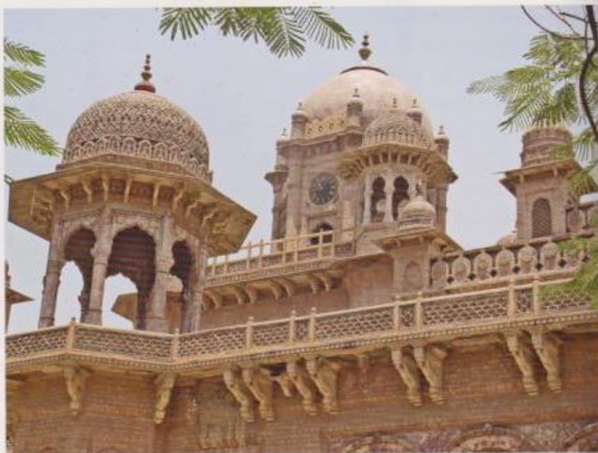
Aitchison College-Main Building
