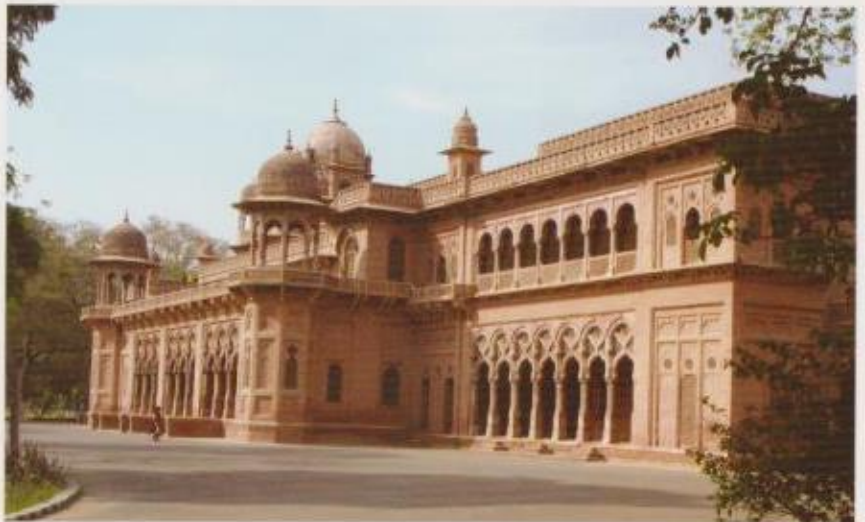
Aitchison College-Main Building
