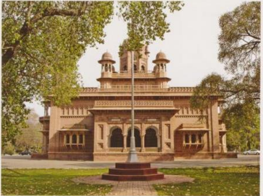
Aitchison College-Main Building
