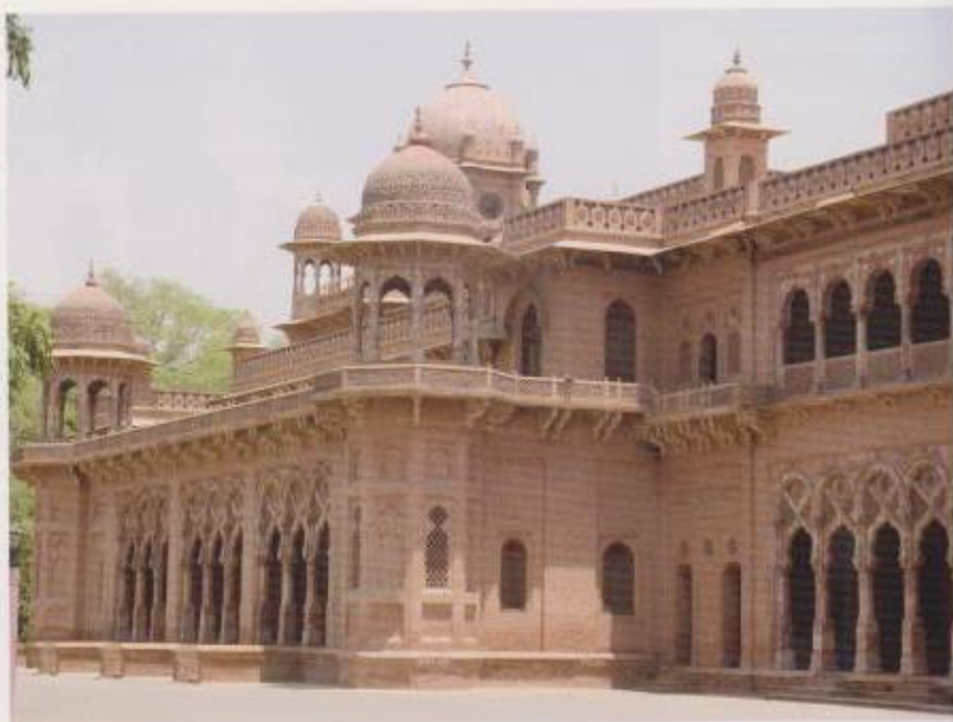
Aitchison College-Main Building
