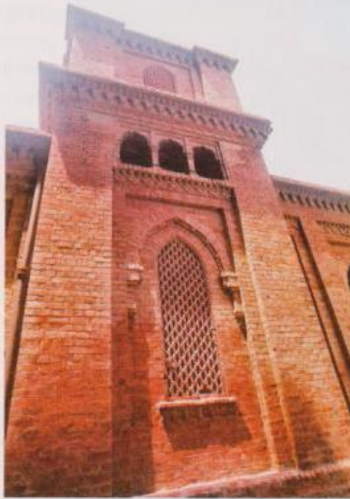
A brickwork feature of the Mayo School of Arts, Workshop Block.
