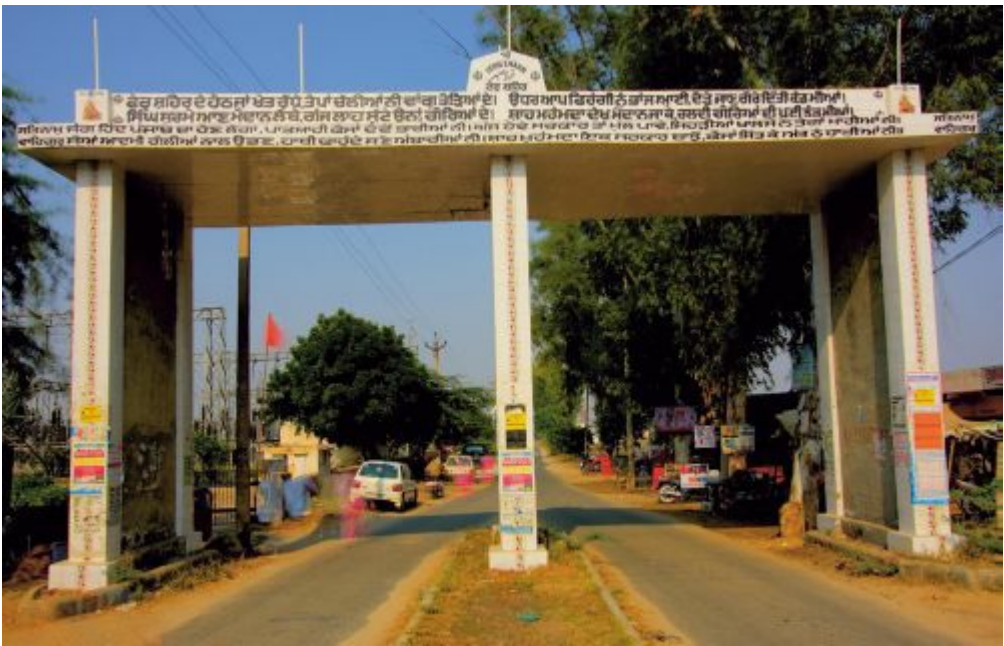
36. An arch built as a memorial to the Battle of Ferozeshah stands at the junction with the NH95 highway. Ahead and to the left, a power substation and various village shops now mar the initial position of the British army and its bivouac during the night of 21 December 1845.
