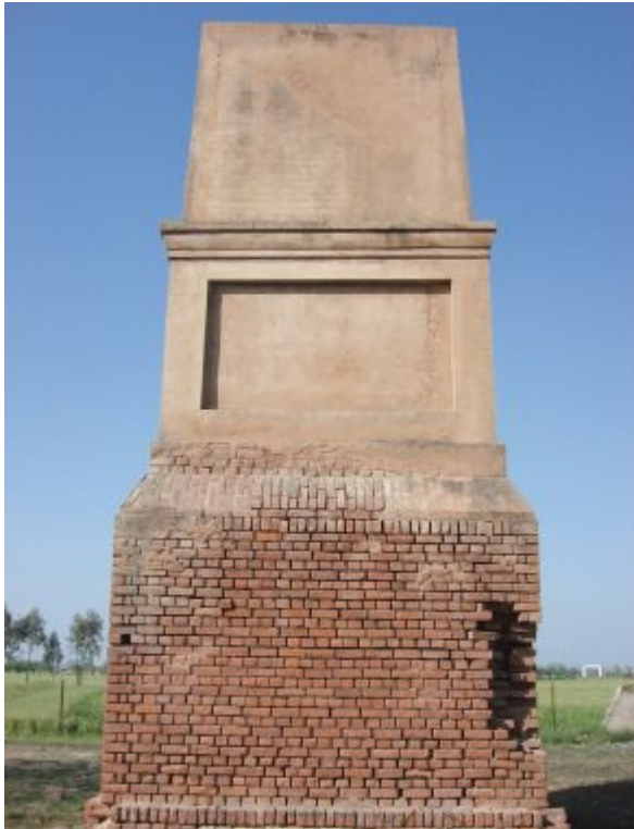
47. The Aliwal monument in the present day. It has lost both its original base and tapering column. The remainder of the monument is heavily altered, suggesting it was at some point rebuilt.
