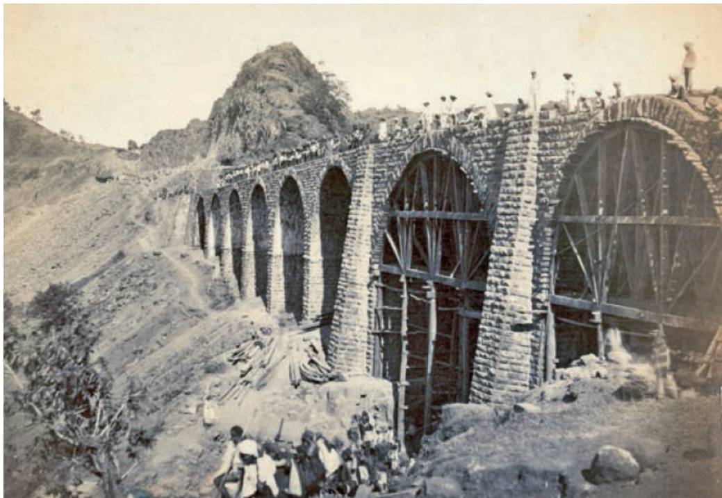
Masons working on a bridge section of Bore ghat incline, between Bombay and Pune, 1855
