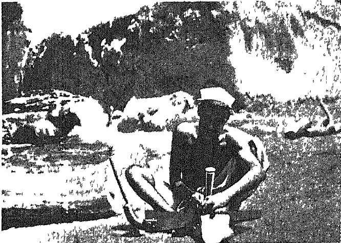
One of the carpenters at work in the lane
