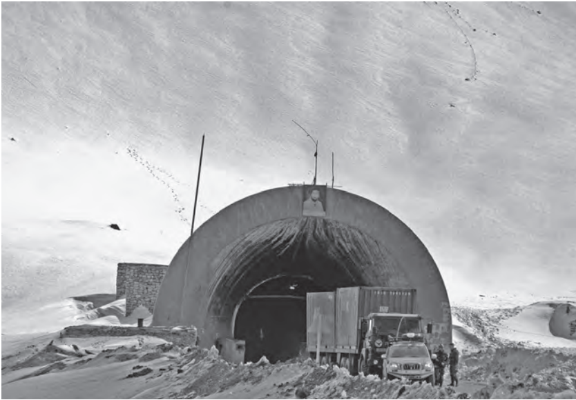
The Salang Tunnel's northern entrance. When completed this 2.6 km (1.6 mi.) tunnel cut travel time from Kabul to Mazar-i Sharif to a single day. However, as the tunnel mouths were built more than 3,000 m (9,842 ft) above sea level, in the winter the approach roads are often blocked.
